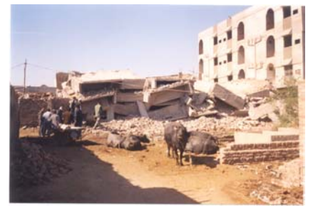
A view of the collapsed block of Ghosia Apartments, Hyderabad
