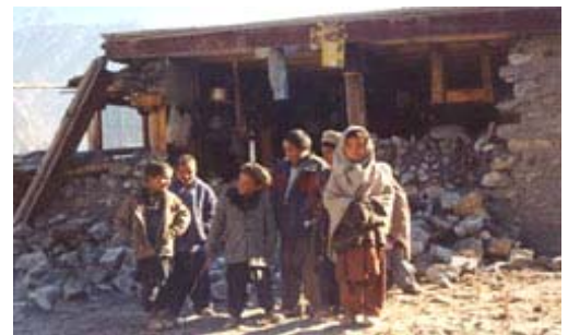
Children outside a collapsed Building Source: Islamic Relief Worldwide
