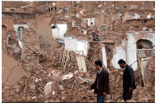
Damaged houses in the city of Zarand.
