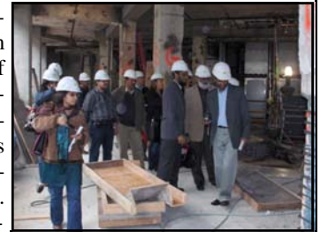
Fig 3: participants tour a retrofit construction site with Holmes Culley Engineers.
