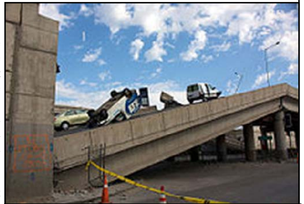
Fig 9: Collapsed Vespucio Norte Express Highway in Santiago.
