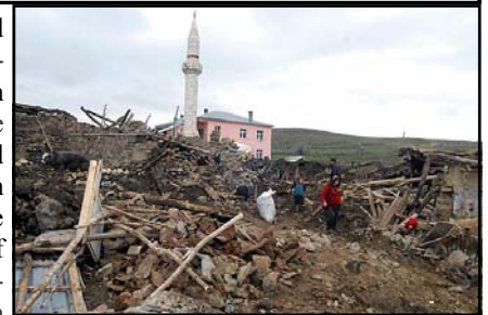
Fig 11: Turkey earthquake destruction
