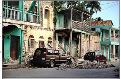
Fig 1: Damaged buildings in Jacmel
