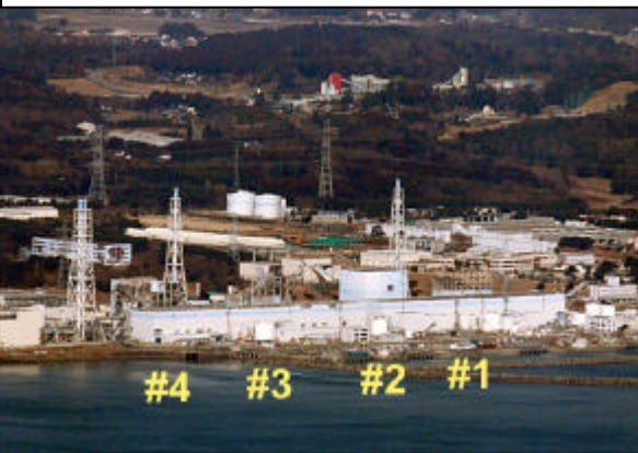
Fig 12: Fukushima Daiichi Nuclear Station showing damaged reactors #1, #3, and #4. Exterior of #2 appears intact although smoke and/or steam has streamed from hole in upper east wall. From ( http://shineyourlight-shineyourlight.blogspot.com/2011/03/japan-one-week-after-
