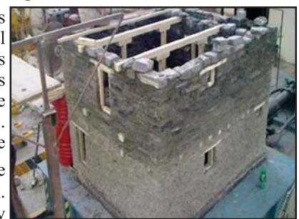
Figure 6: Construction of 1/3rd model of Hunza Ha on the shake table.
