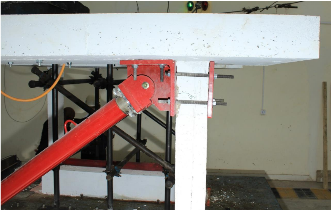
Fig. 15 Crack in the column of BRB strengthened frame at 375% level of test run
