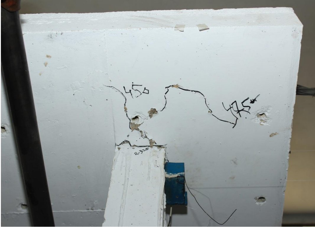
Fig. 16 Cracks in the overhanging part of top slab in control frame
