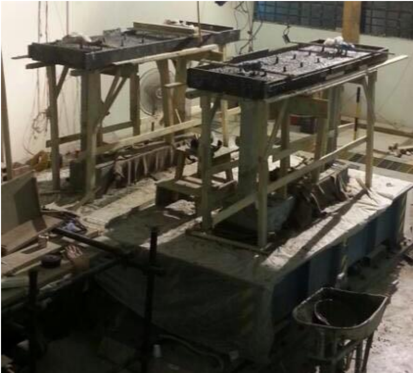
Fig. 8 Casting of top slab of frames
