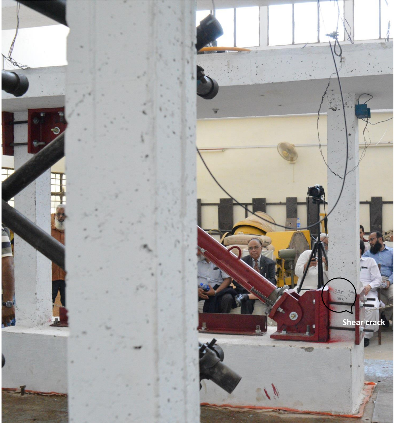
Fig. 11 Shear crack in the column of BRB strengthened frame at top of end plate
