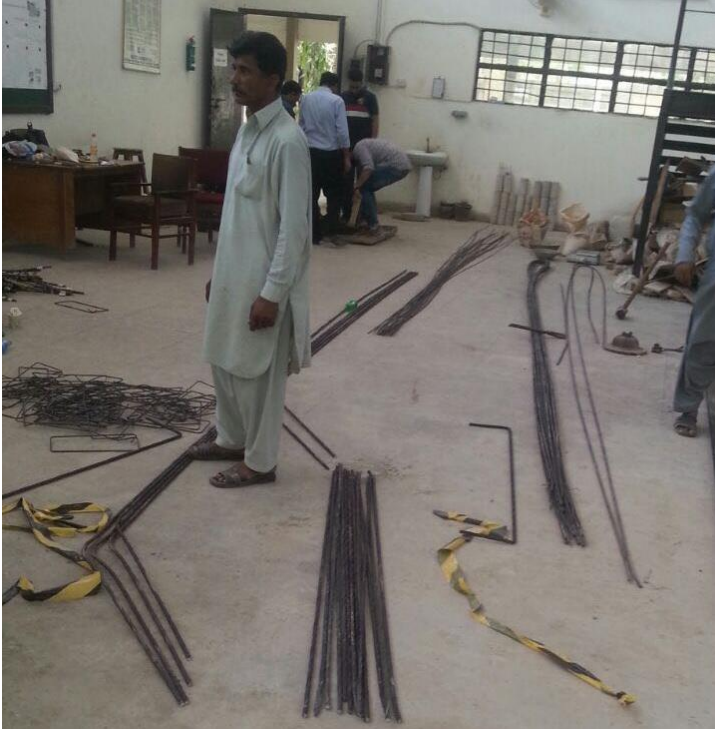
Fig. 5 Cutting and bending of steel for frames
