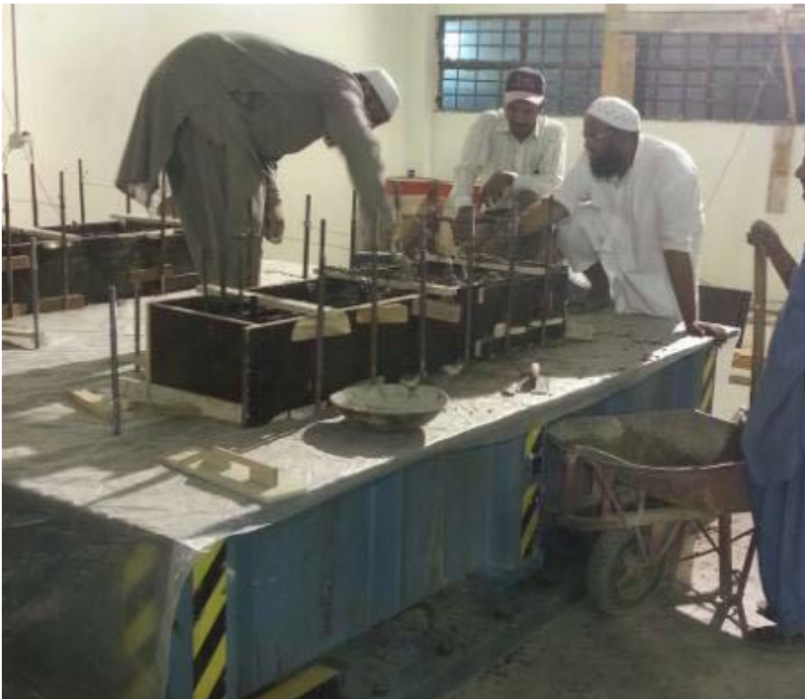
Fig. 6 Casting of foundation beam
