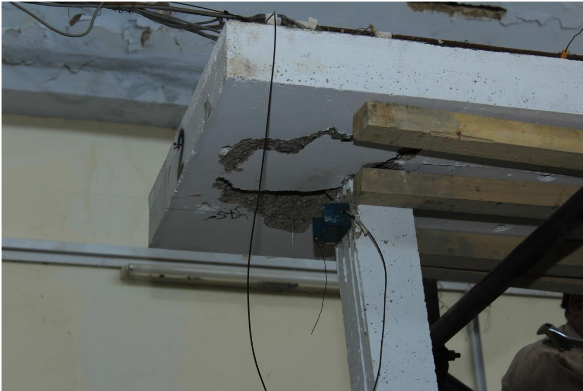
Fig. 17 Damaged portion of top slab for control frame
