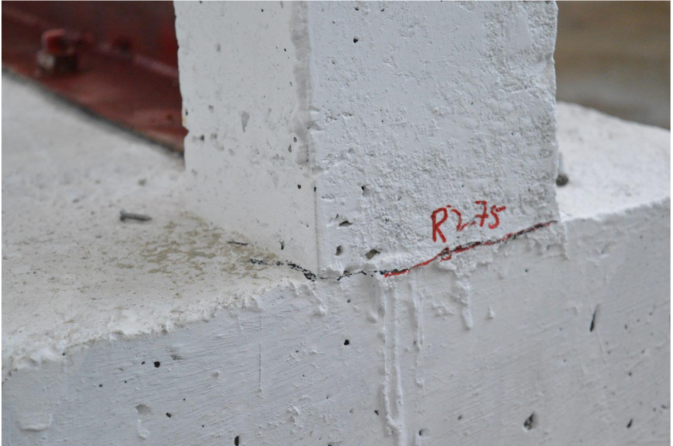
Fig. 10 First level crack in the column of control frame
