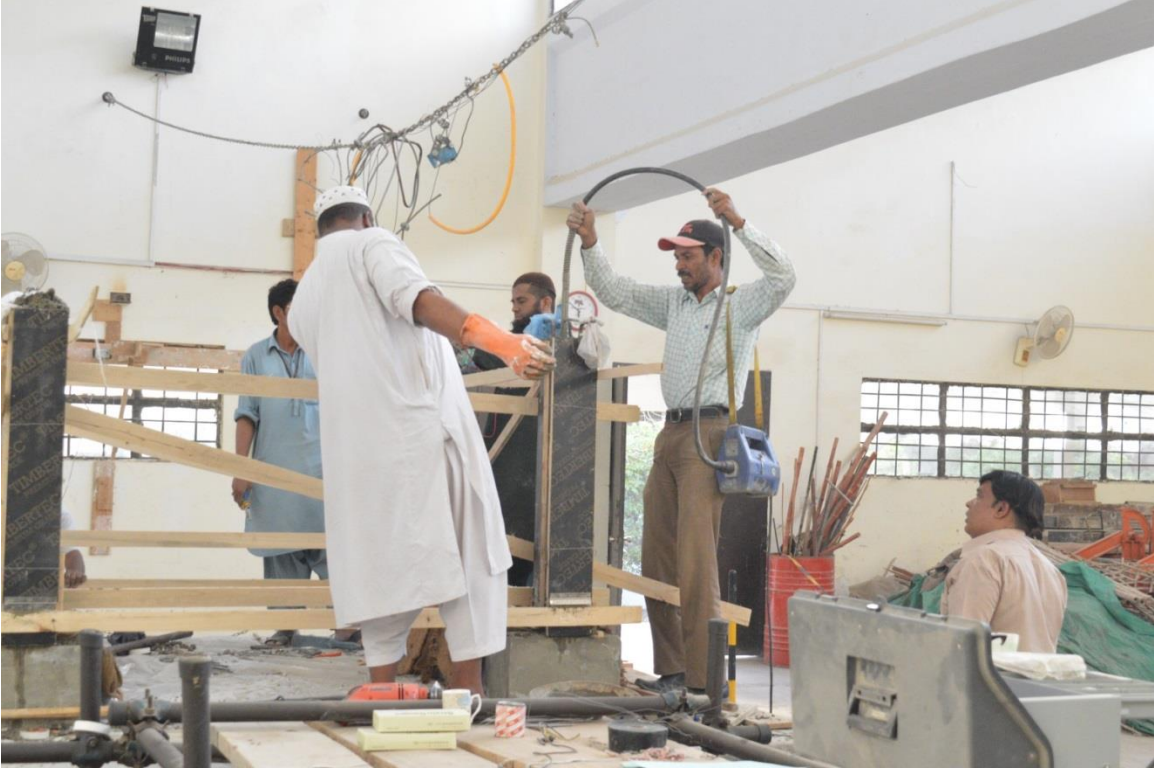
Fig. 7 Concreting of columns
