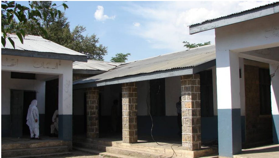
Figure 1. View of the case-study school building before retrofitting.
