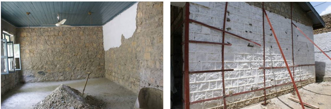
Figure 15. Preparation of surface inside school (left); installation of steel straps (right)
