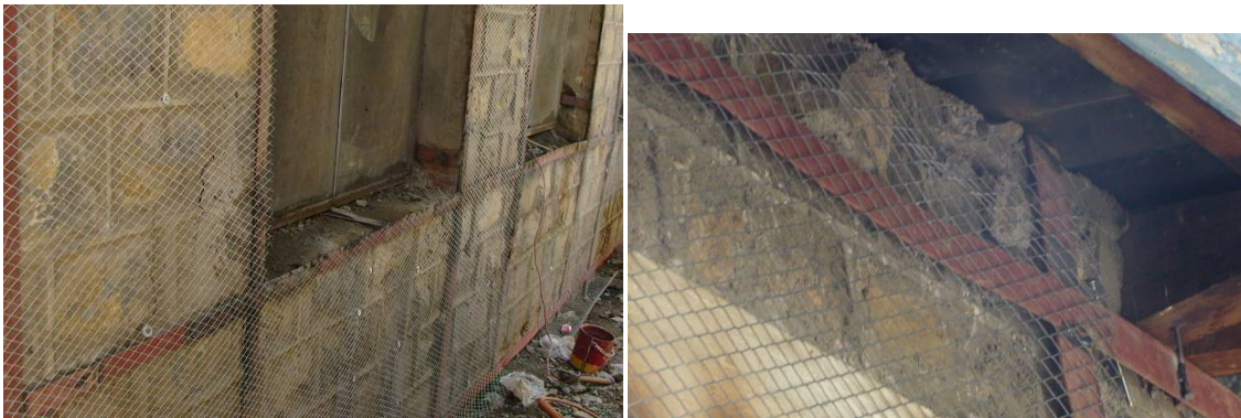
Figure 11. Installation of vertical and horizontal metal strips
