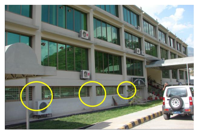
Figure 12. Captive columns at ground storey
