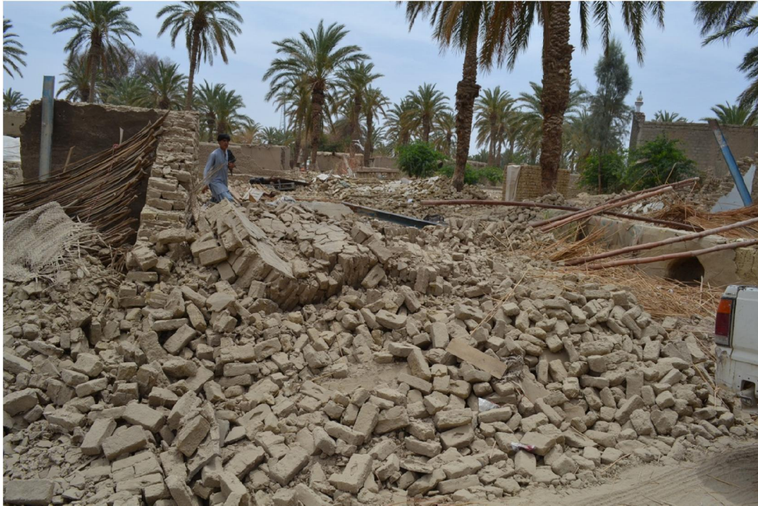
Fig. 8 View of damages in West Zawag
