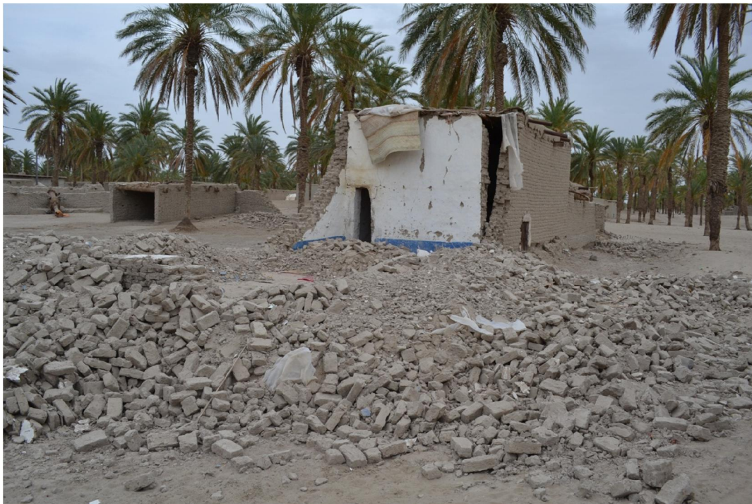
Fig. 11 Damaged adobe houses in Kili Kallag
