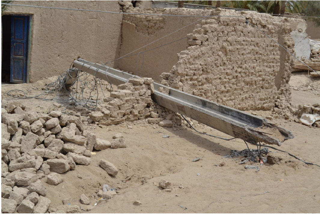
Fig. 4 Broken electricity poles in West Zawag
