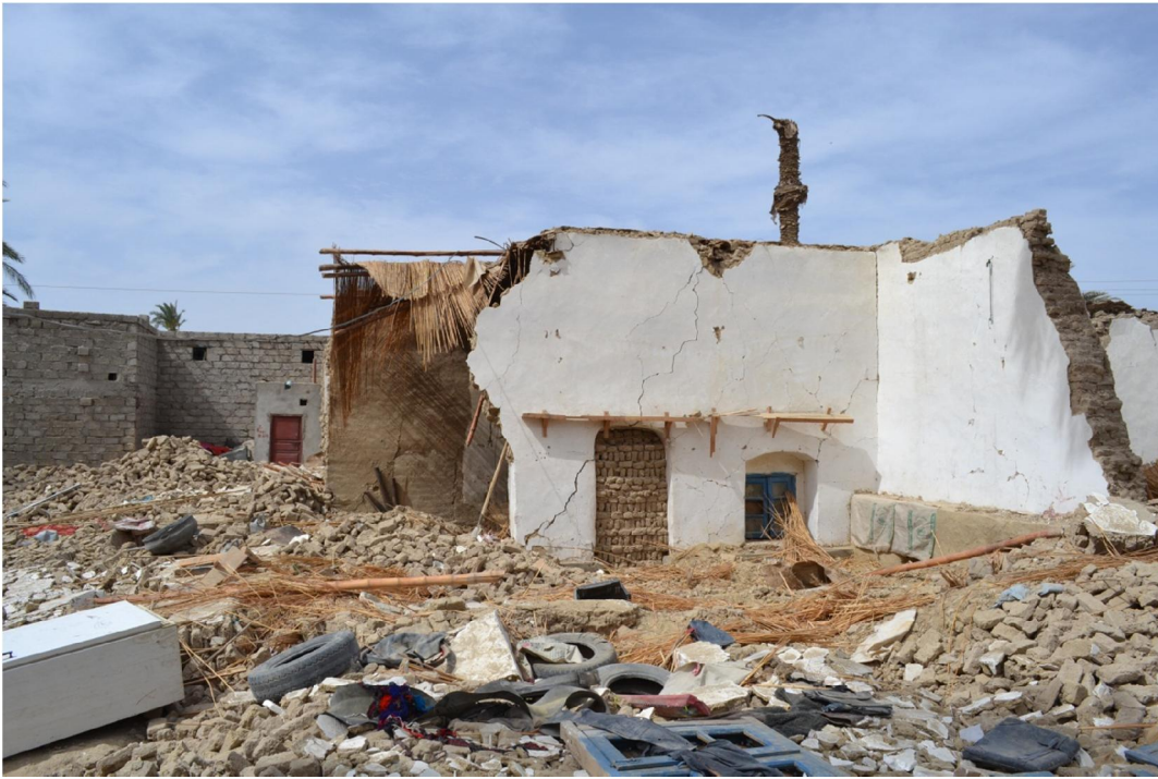
Fig. 7 Damaged adobe buildings in East Zawag
