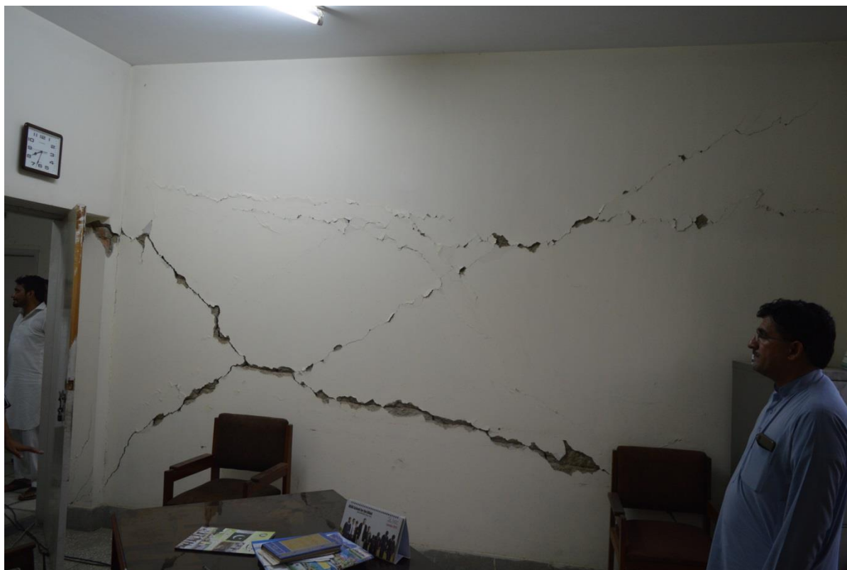
Fig. 6 Wall cracks in Radio Station building at Mirpur
