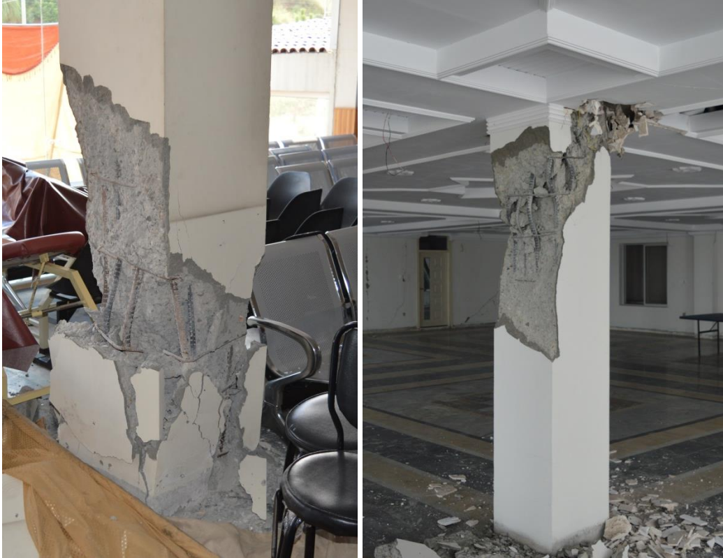
Fig. 13 Damaged columns in Ahsan Medical Complex building
