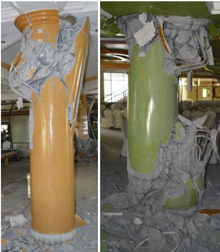
Fig. 12 Column damages in Gulshan-e-Jabeer
