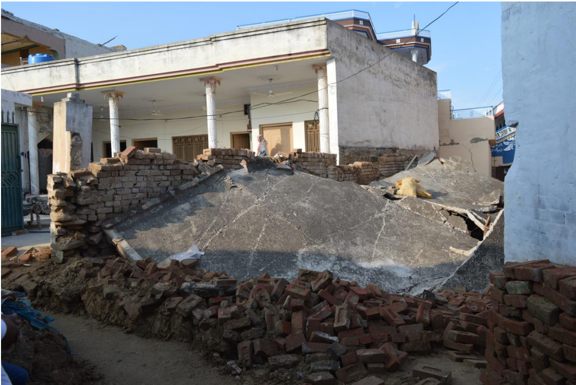
Fig. 9 Collapse of cattle shed
