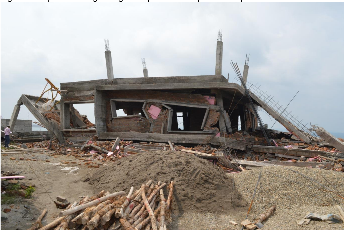
Fig. 15 Collapse of a storey of an under construction building
