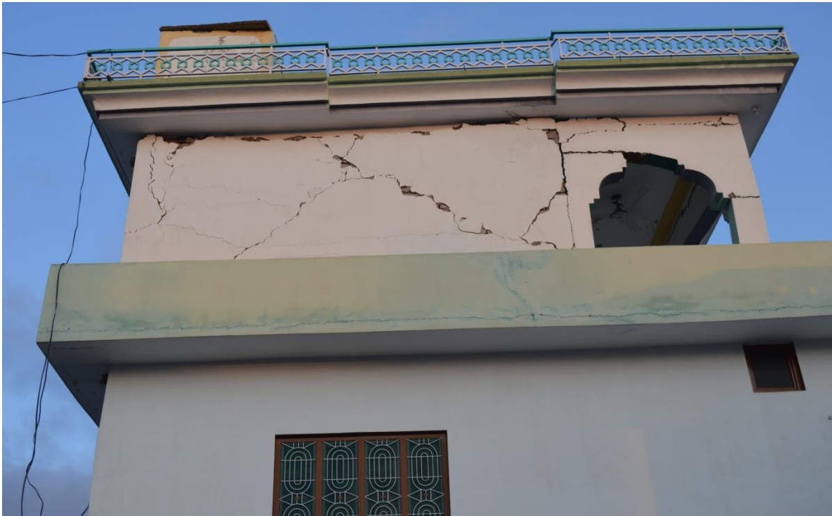
Fig. 7 Residential building with diagonal wall cracks
