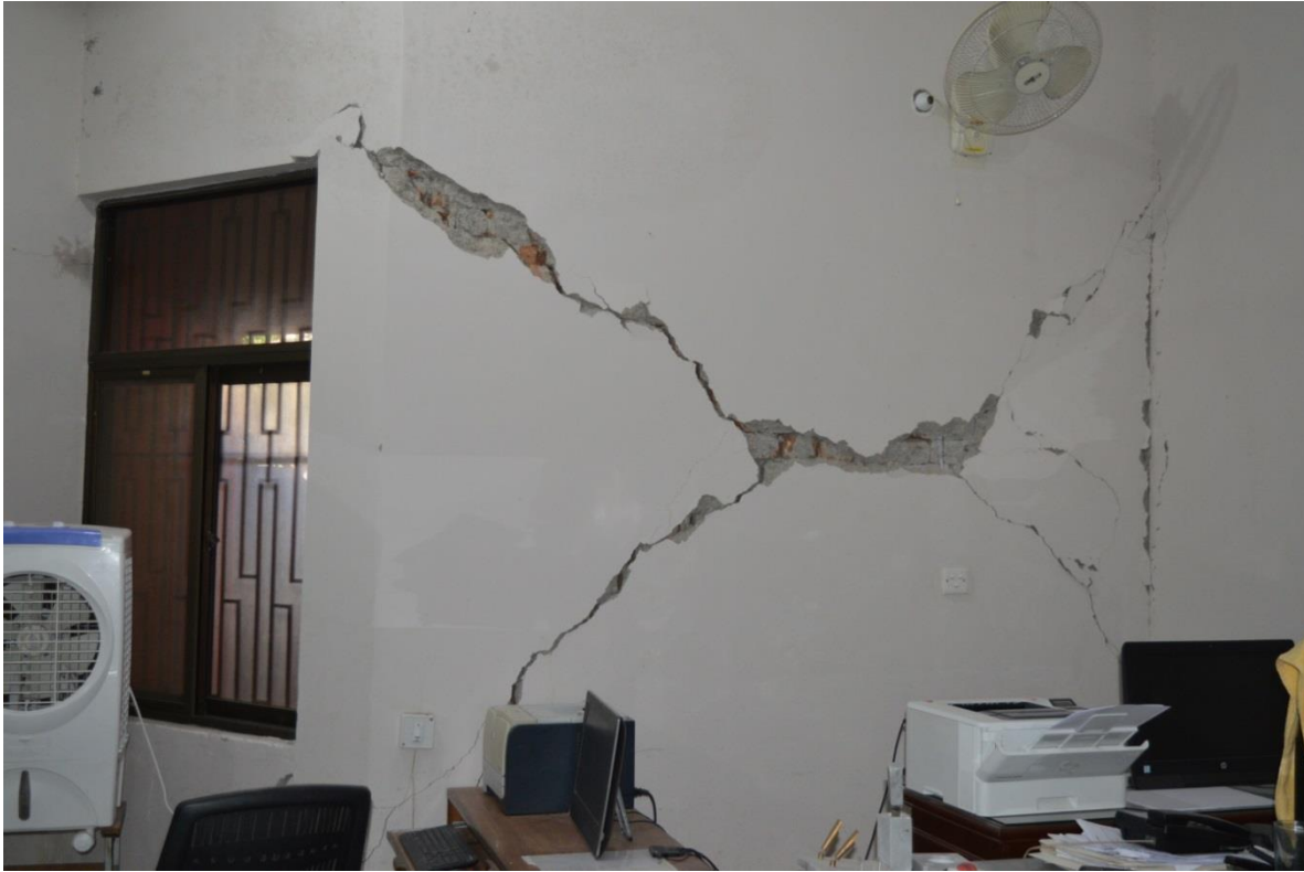
Fig. 4 Cracks in walls in Admin building at MUST
