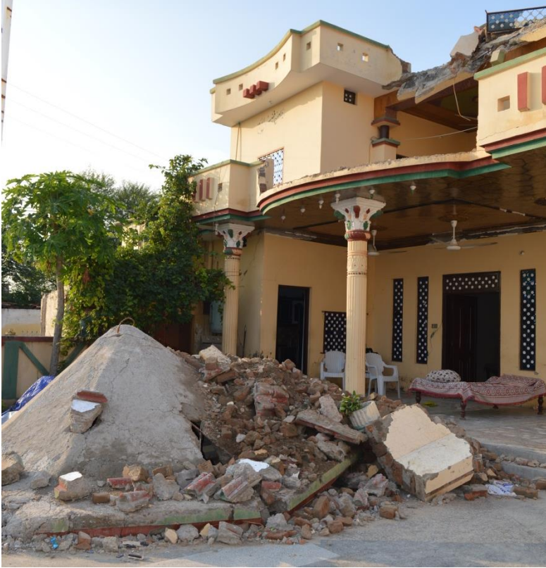
Fig. 8 View of fallen circular roof of stair tower
