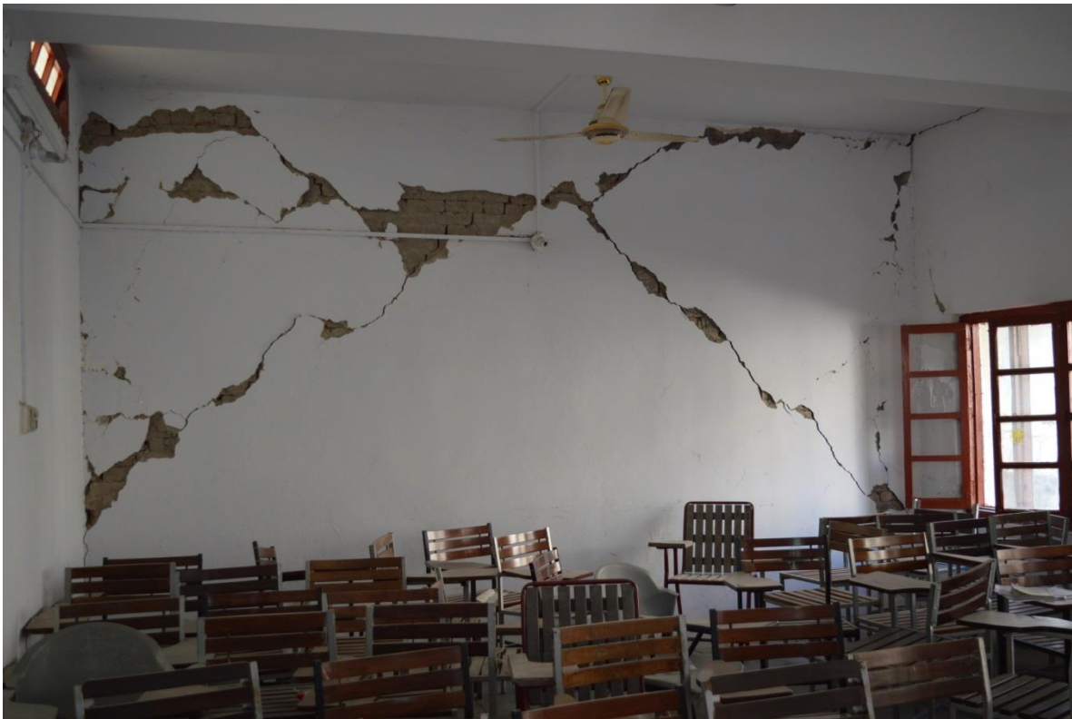
Fig. 5 In-plane shear cracks in classroom in Home Economics Department building
