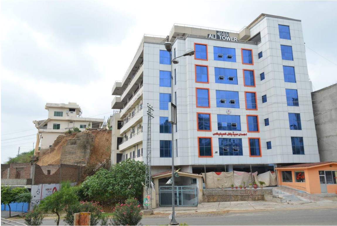
Fig. 11 View of Ahsan Medical Complex building
