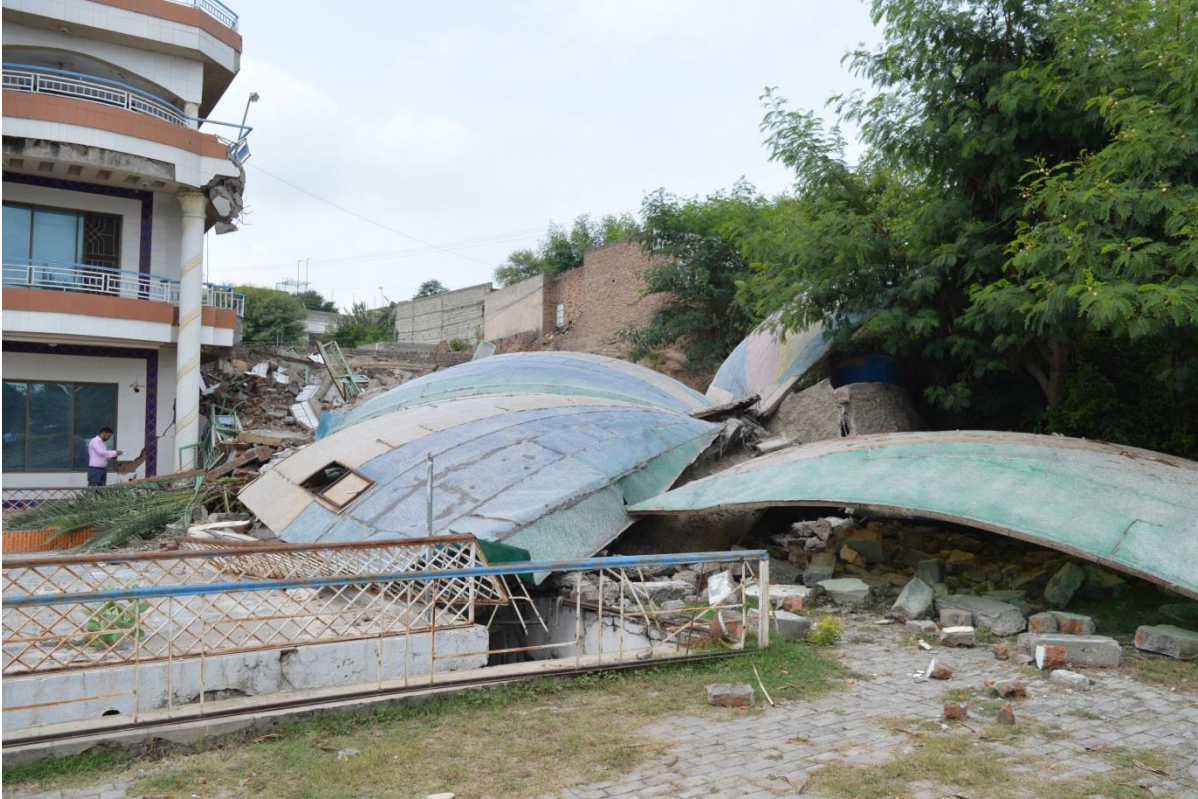
Fig. 14 Collapsed building during 24 Sep 2019 earthquake in Mirpur
